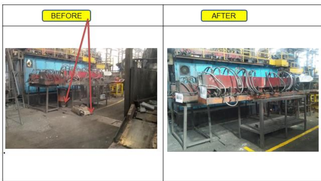
Fig2 Unwanted Material Removed
